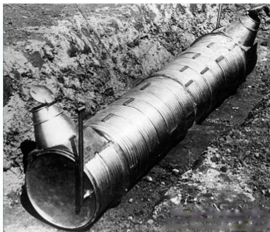
Russian buried KVS-U prefabricated buried corrugated steel shelter
